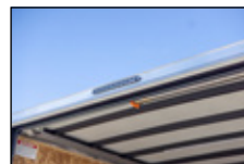
Bowed Roof Crossmembers
